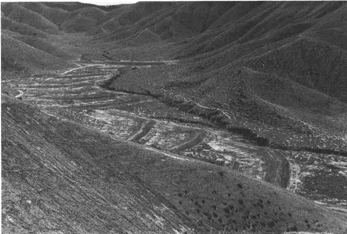
Elephant Skin Wash salinity control verification project near Montrose, Colorado.
